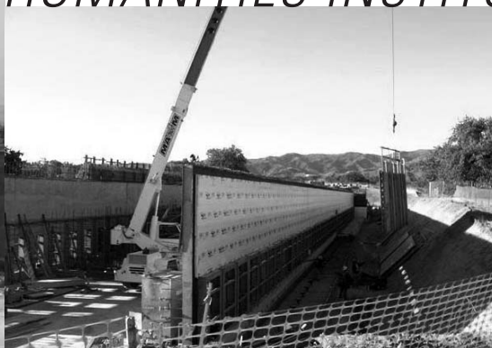
Nitrate vaults under construction.
